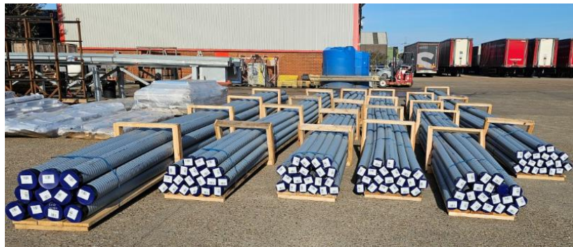
Figure 25 – Heat network pipe bundles
