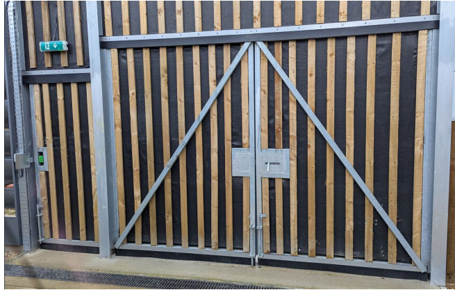
Figure 3. Gaps at top and bottom of single and double leaf gates covered; plate fixed next to push-lever on single leaf gate next to louvre
