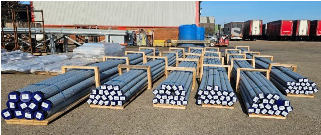
Figure 25. Heat network pipe bundles
