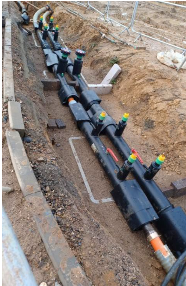
Figure 40. DRP valves laid prior to completion of chamber housing
