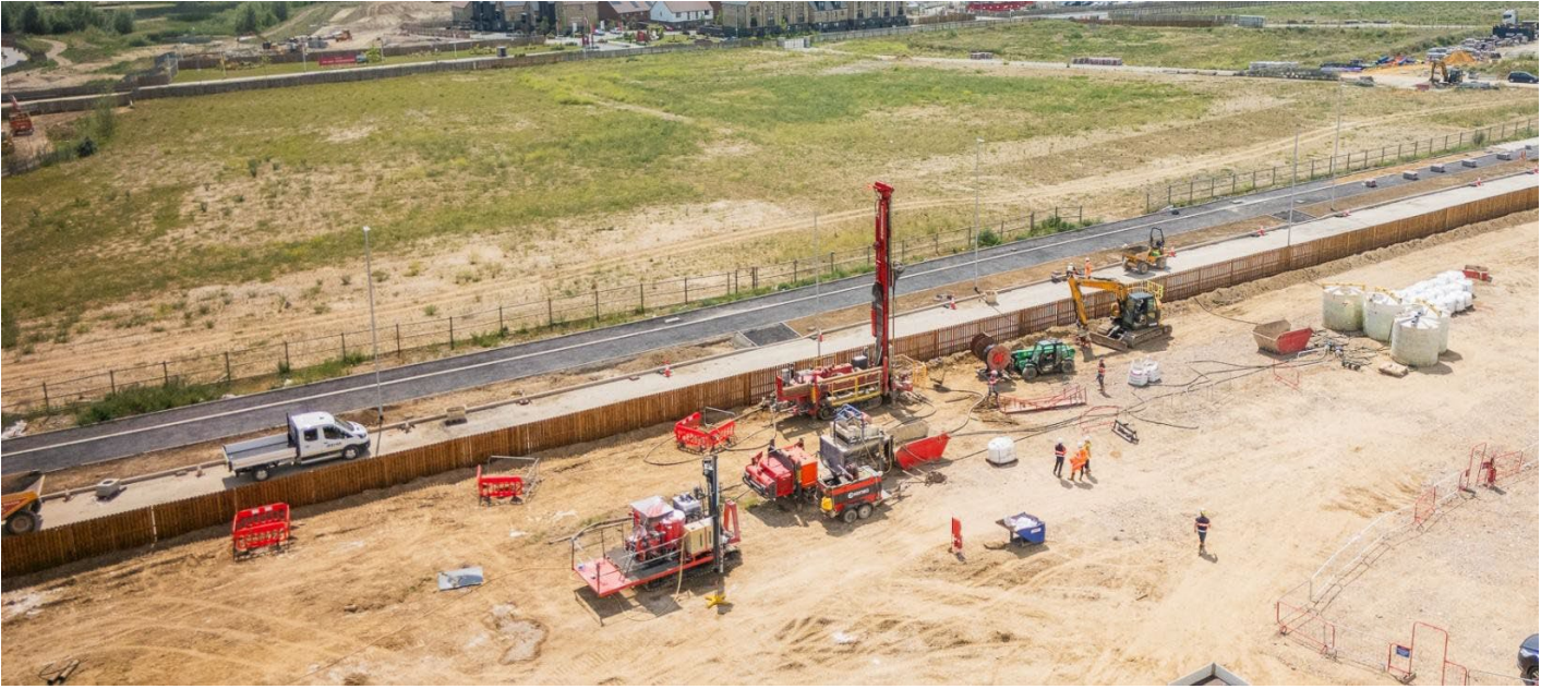
Figure 11. Site during drilling of Boreholes
