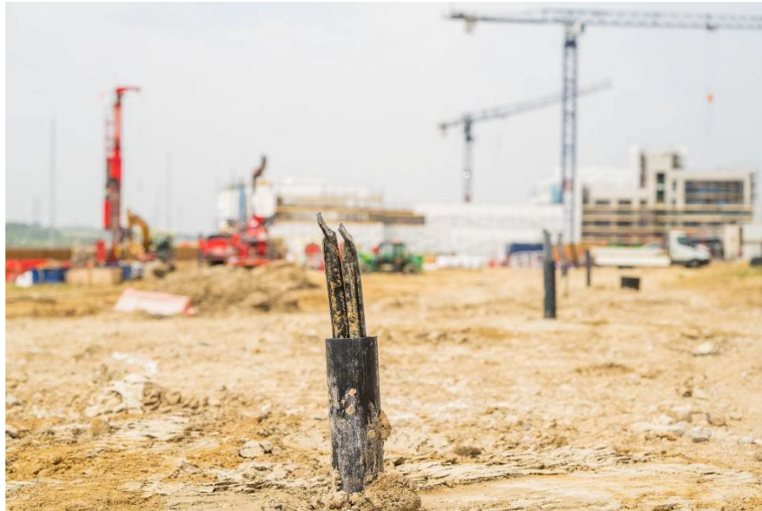
Figure 8. Boreholes left with sealed ends
