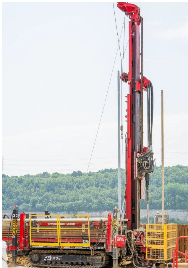
Figure 7. Example of typical rig used for drilling
