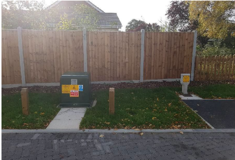
Figure 33. An example of how a small above ground installation should be finished
