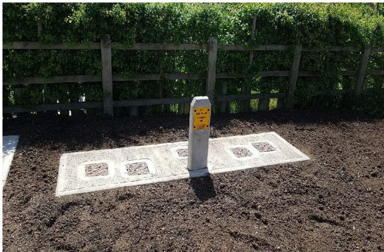
Figure 34. An example of how the valve nest should be finished
