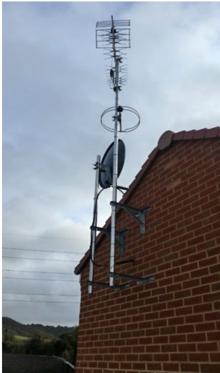
Figure 25. E.4 satellite dish, DVB-T and DAB antenna installation on OSCP/substation building
