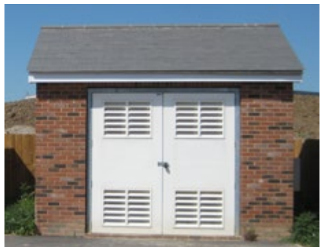
Figure 24. E.3 OSCP building
