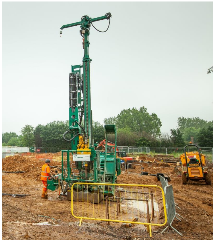
Figure 2: Example of typical rig used for drilling
