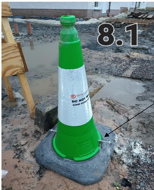
Figure 3: Example of cone secured to borehole top to assist in preventing damage (e.g. by later civils works)
