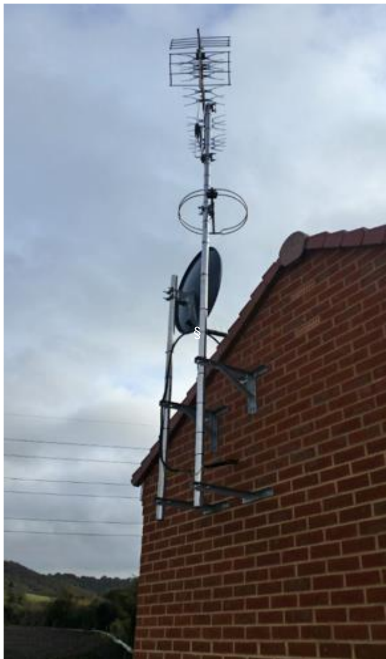
Figure 26 – E.4 satellite dish, DVB-T and DAB antenna installation on OSCP/substation building
