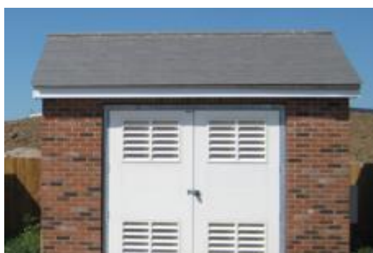
Figure 25 – E.3 OSCP building
