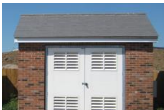
Figure 25 – E.3 OSCP building
