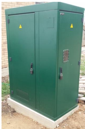
Figure 24 – E.1 voice and data (non-FIRS) cabinet
