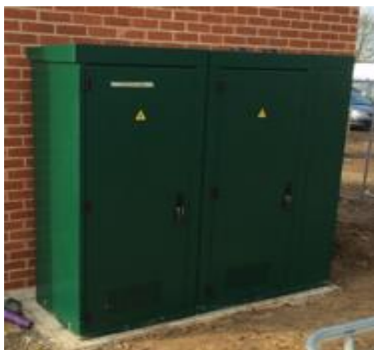
Figure 23 – E.2 voice and data with FIRS cabinet
