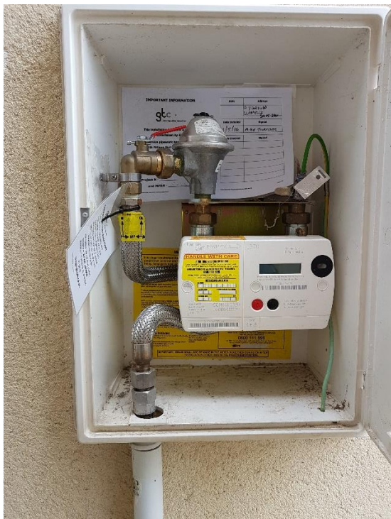
Cavity meter box with braided steel flexible hose Information label within meter box
