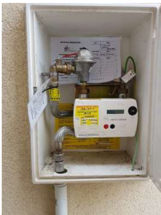
Cavity meter box with braided steel flexible hose box
