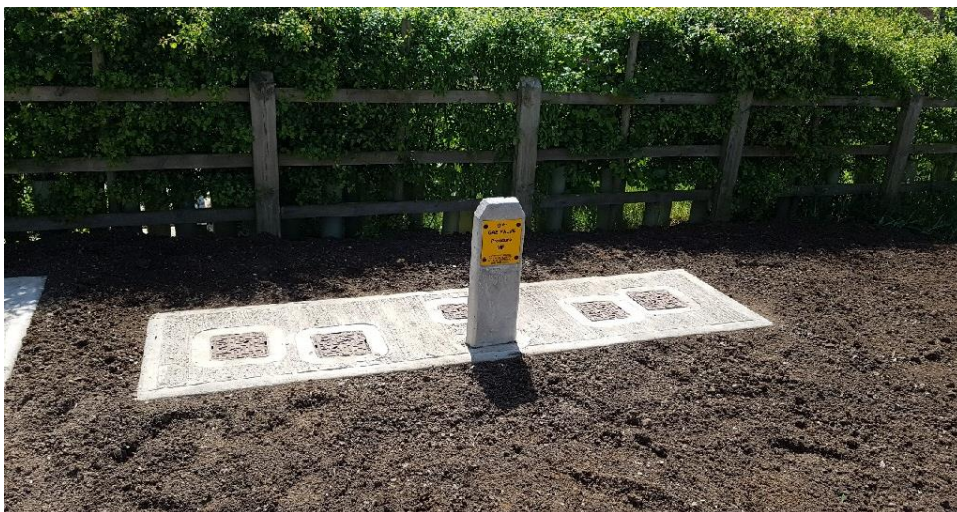
Figure 34 – An example of how the valve nest should be finished
