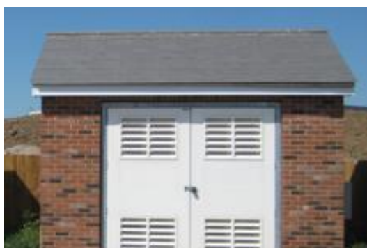
Figure 25 – E.3 OSCP building
