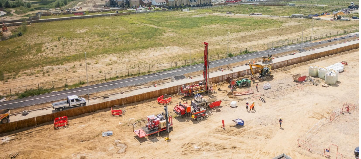
Figure 11: Site during drilling of Boreholes
