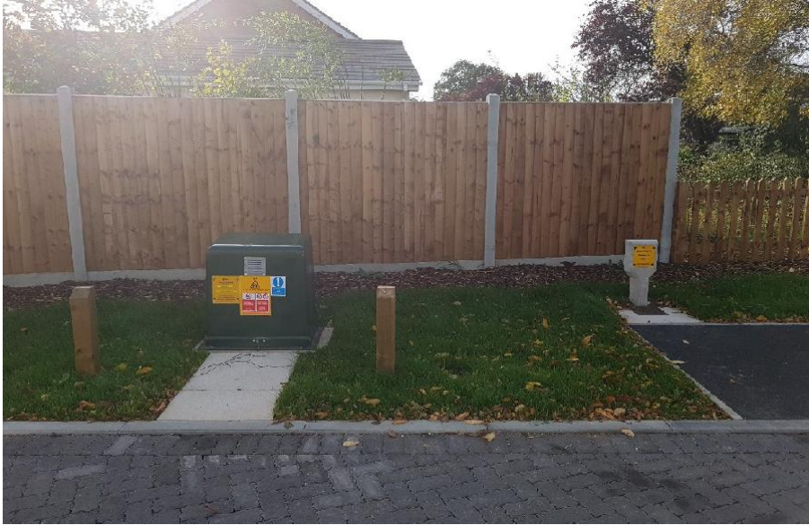
Figure 33 – An example of how a small above ground installation should be finished
