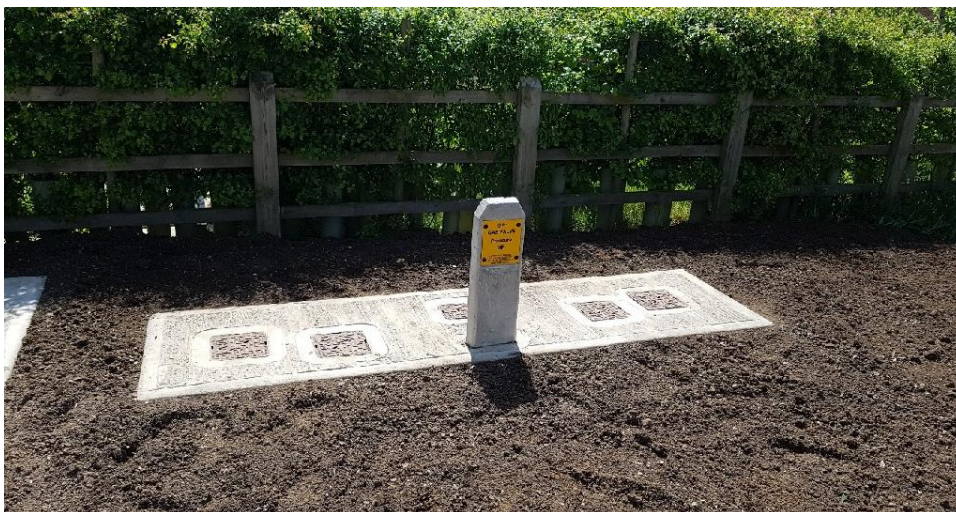
Figure 34 – An example of how the valve nest should be finished
