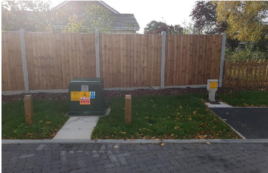
Figure 33 – An example of how a small above ground installation should be finished
